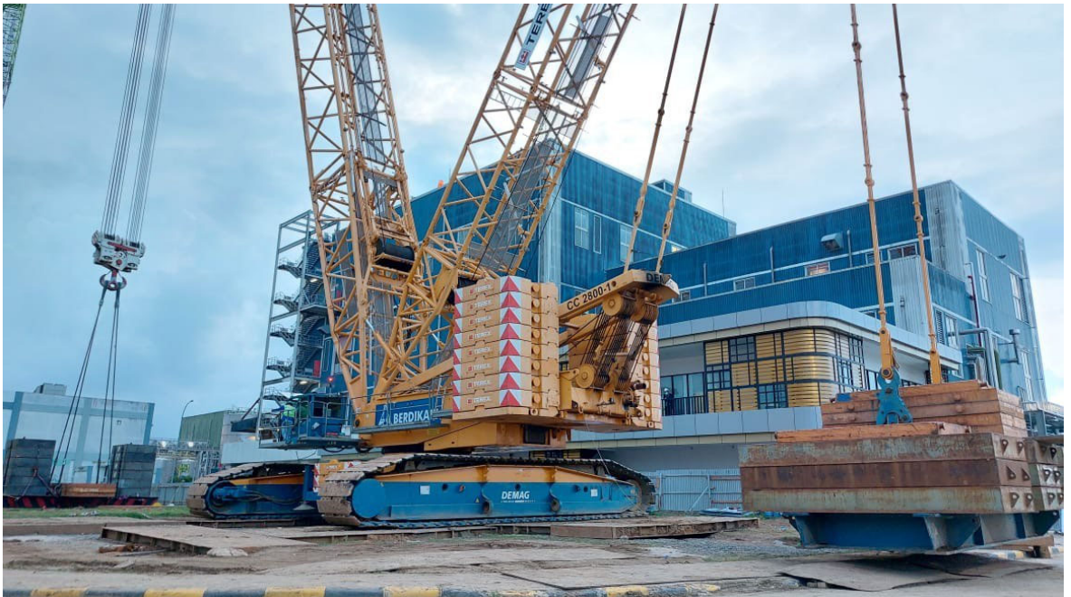
Gambar 4. Heavy Lift Crawler Crane
