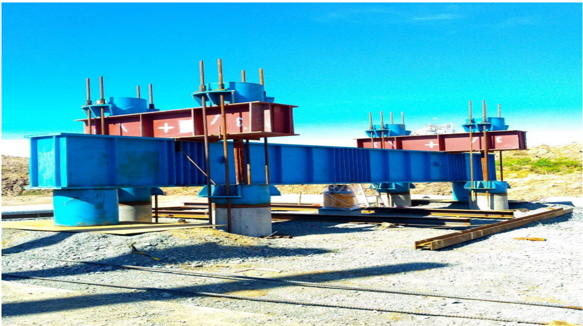
Gambar 6. Loading Test Equipment
